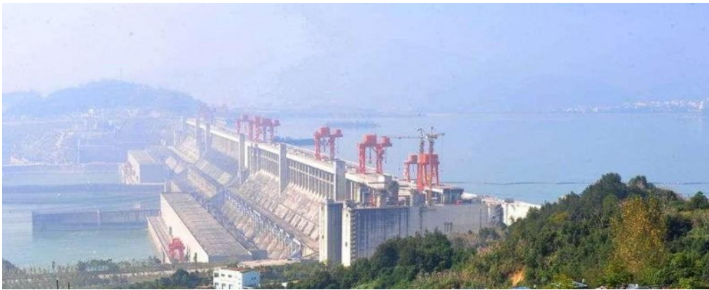
Figure 8. Three Gorges Dam
